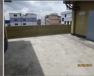
External photo(s) of the production unit(s) Rooftop.JPG
